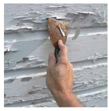
This is a **HAZARD** that can cause lead poisoning because the bottom layers of paint may contain lead, even if the surface has been repainted with lead-free paint.
