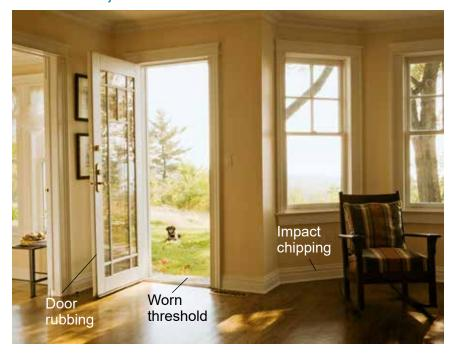
Check all surfaces for chipping and peeling paint. Look for paint chips on the floor and in the carpet. Look for impact chipping at corners of door frame, baseboard and walls. Look for rub or scrape marks on door edges.
